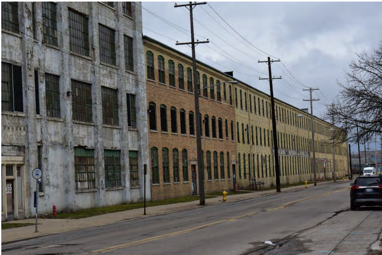
5- and 3-Story Buildings Looking North
