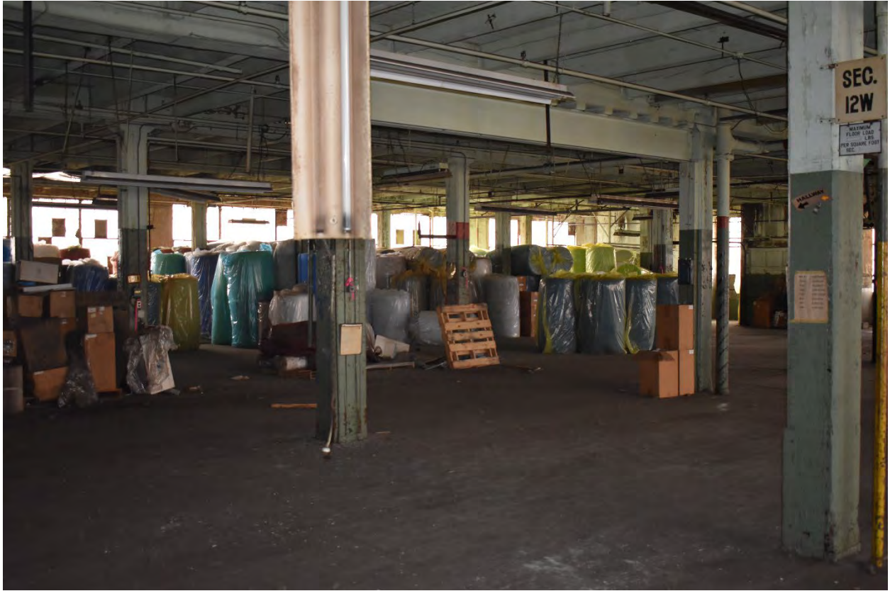
Interior view of the 3-Story Building
