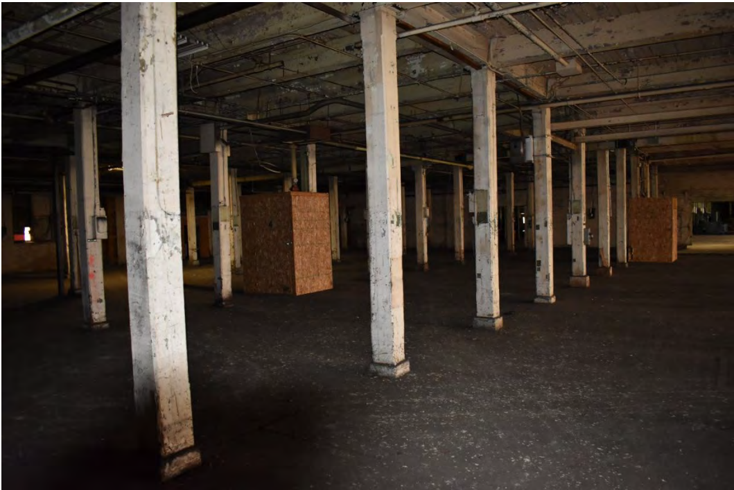
Interior view of the 3-Story Building
