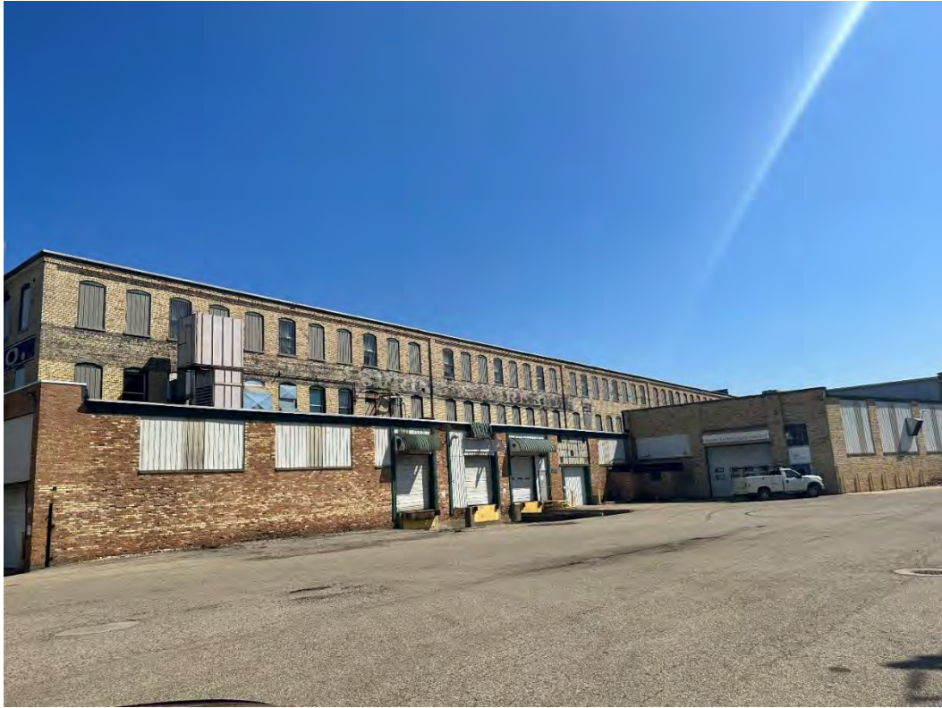
View looking SE from the NW end of the Three-Story Building
