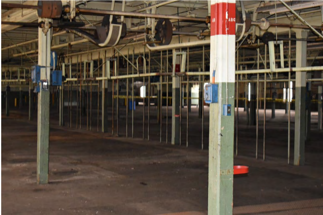
Interior view of the 3-Story Building
