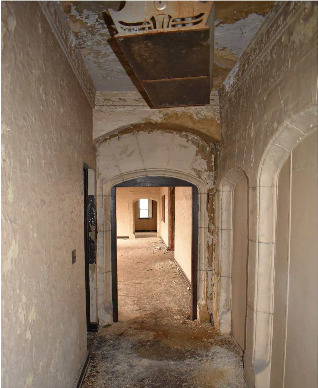
Interior view of the 5-Story Building
