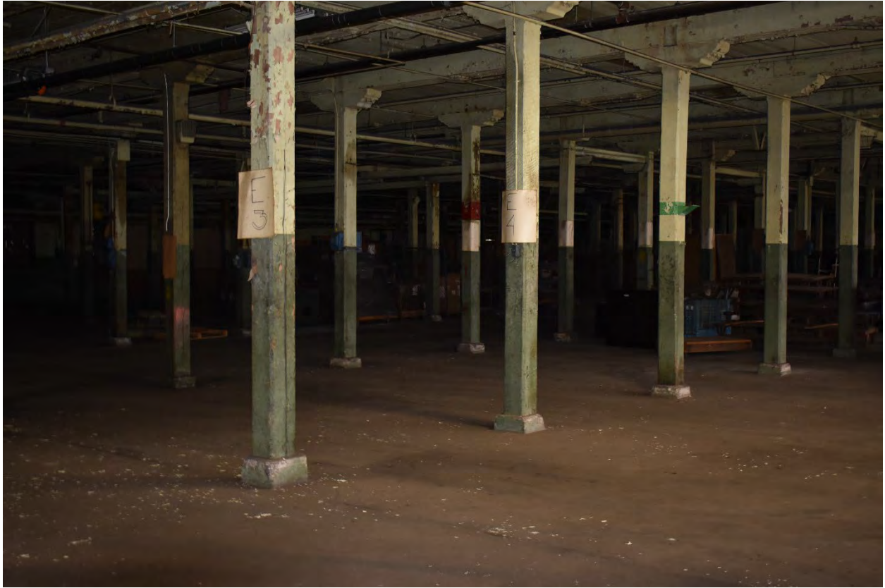
Interior view of the 3-Story Building
