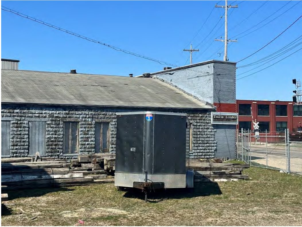
View looking toward the NEC of the North Commercial Site
