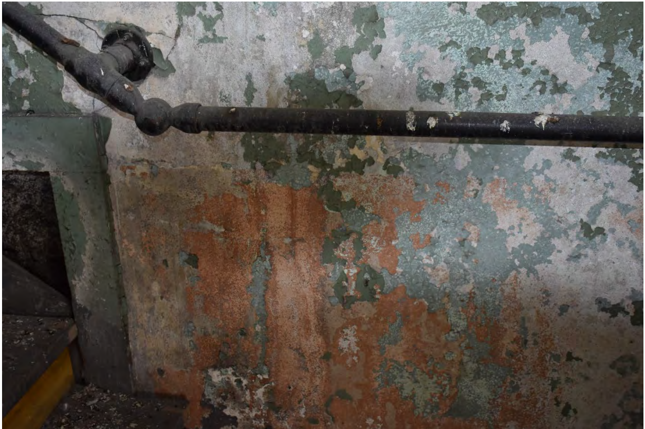
Interior view of the 3-Story Building
