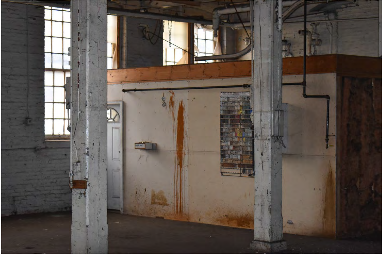
Interior view of the 3-Story Building
