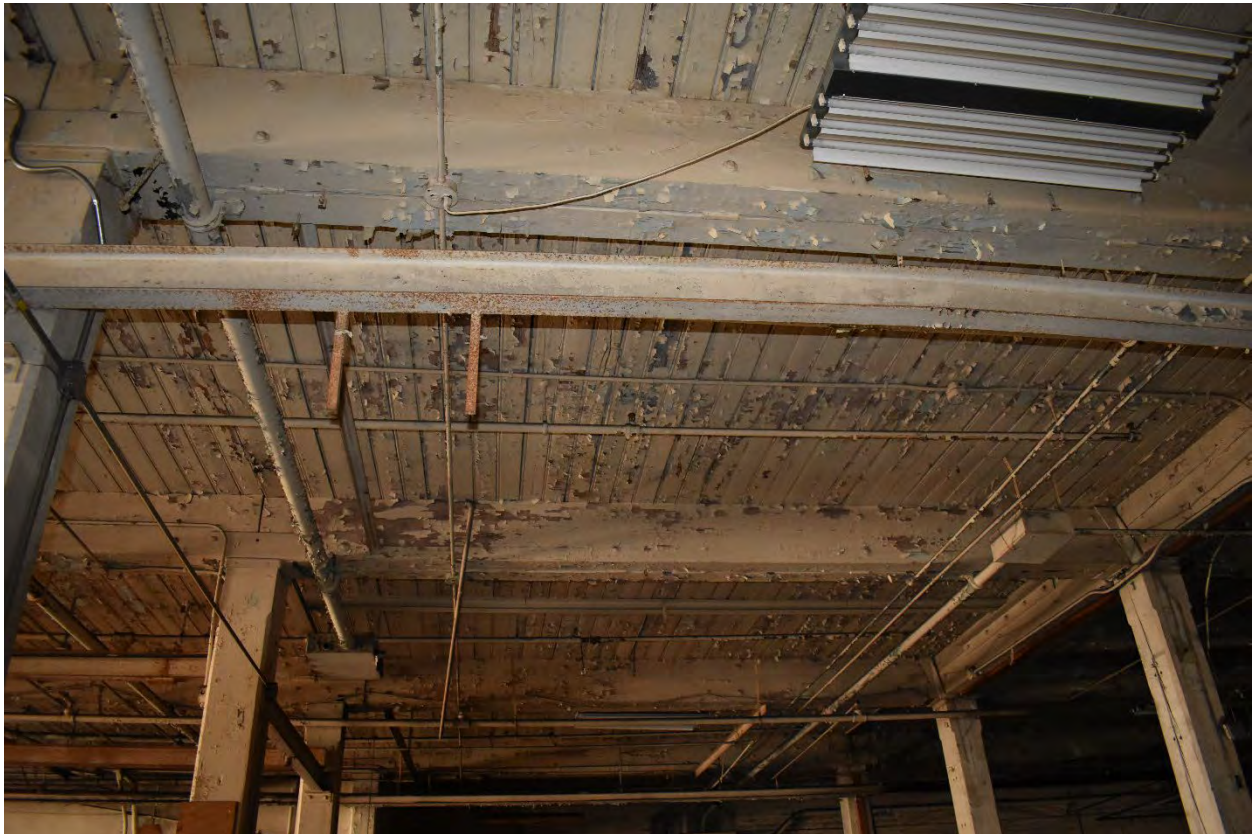
Interior view of the 5-Story Building
