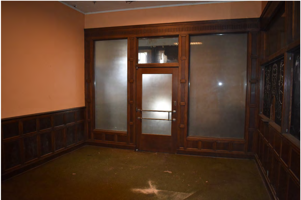
Interior view of the 5-Story Building
