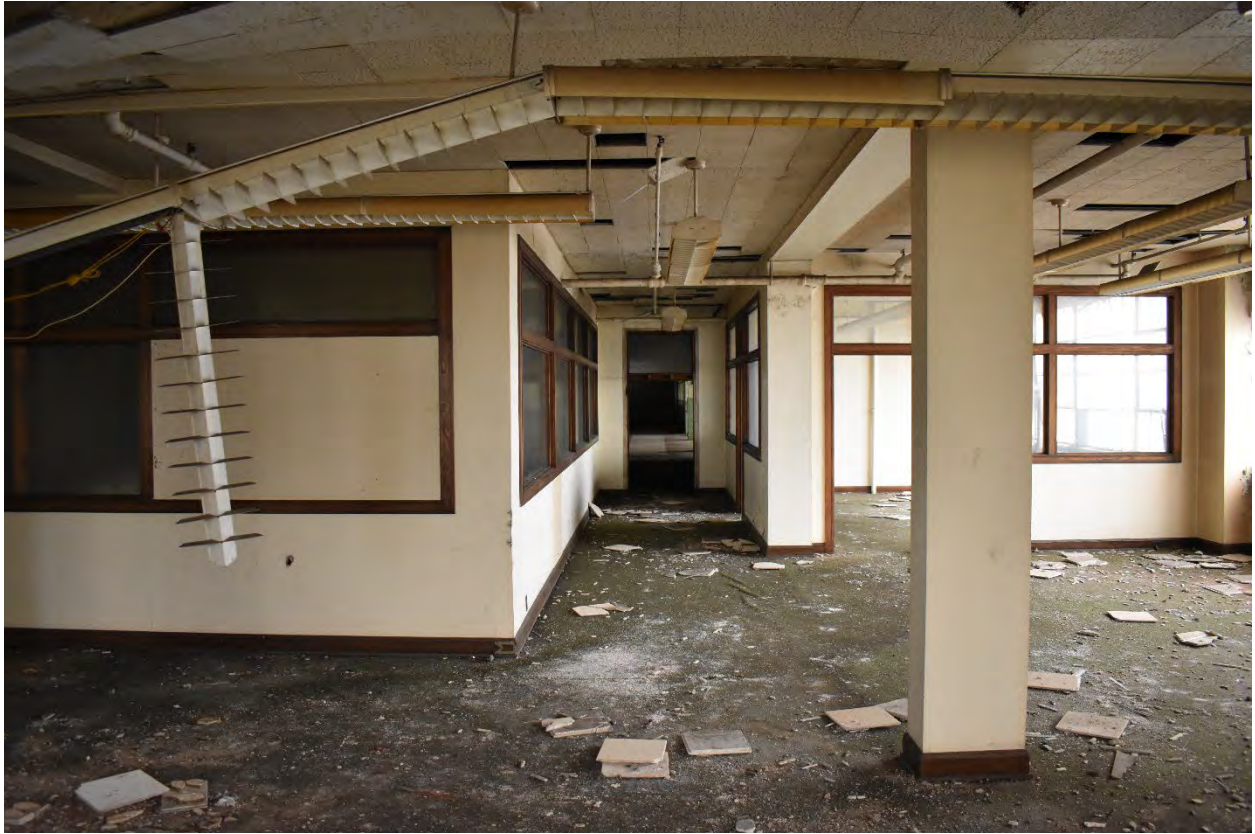
Interior view of the 5-Story Building
