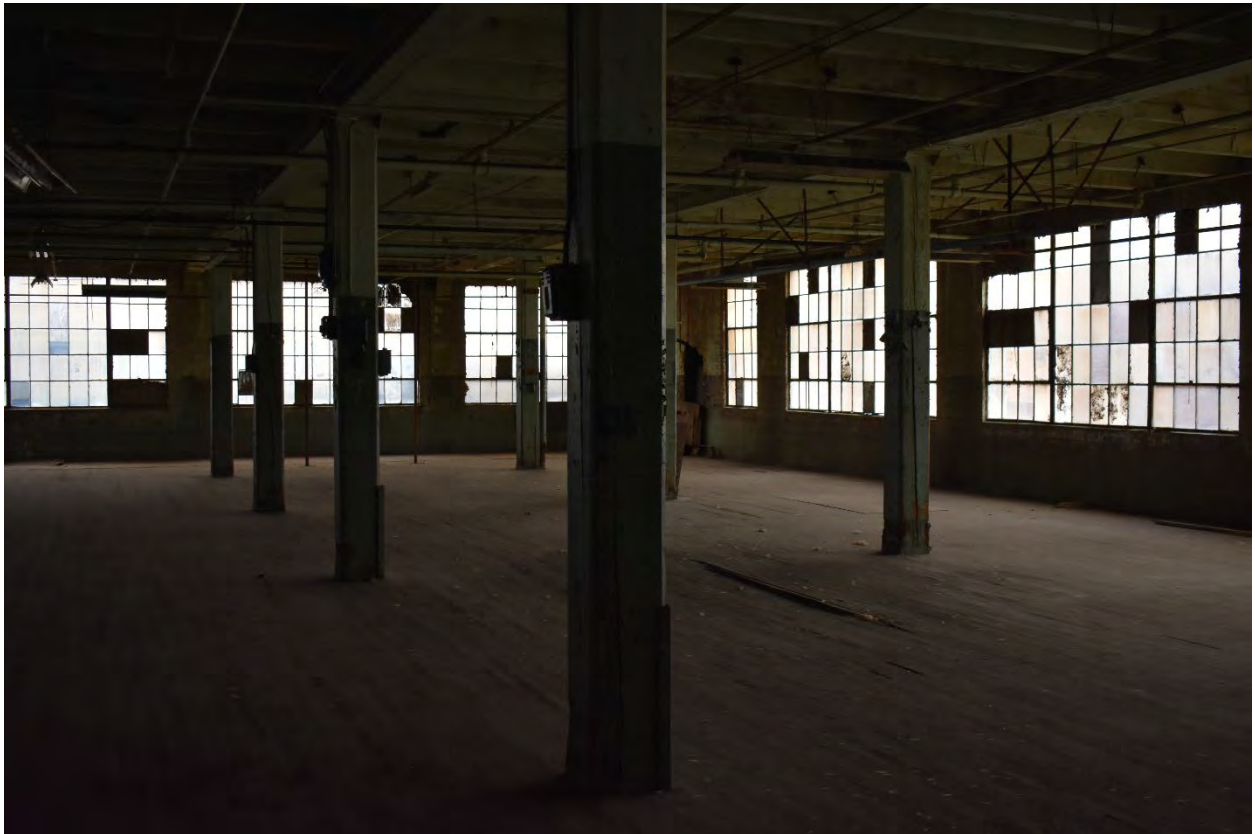
Interior view of the 5-Story Building
