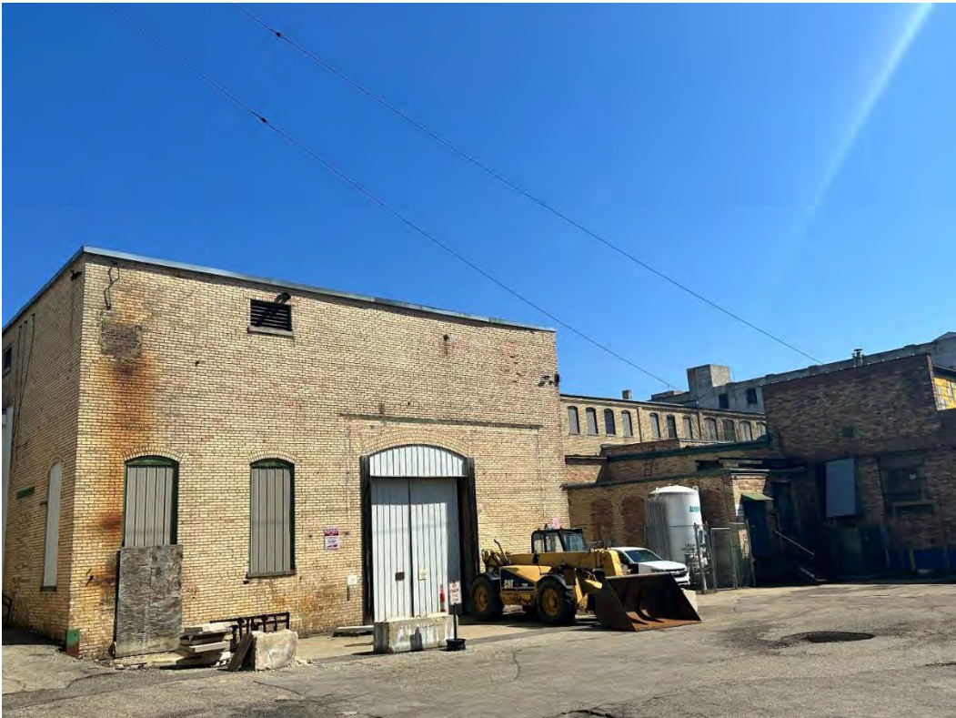
View of the Boiler House building from the west
