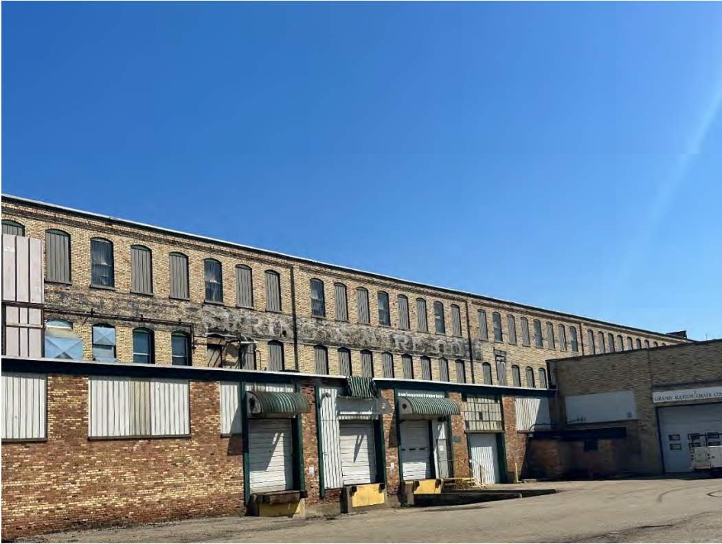
SE view of the west side of the 3-Story Building
