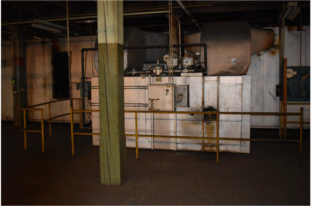
Interior view of the 3-Story Building
