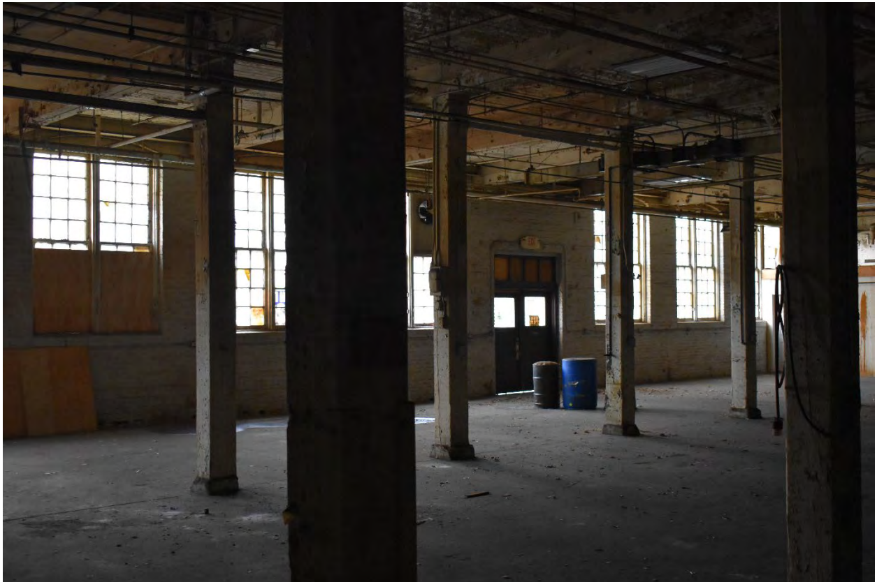
Interior view of the 3-Story Building
