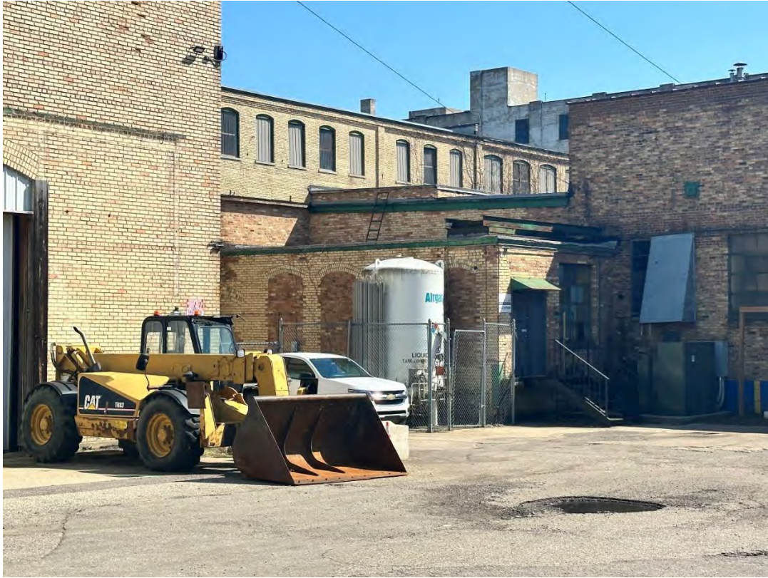
Looking SE Near the Boiler House Building
