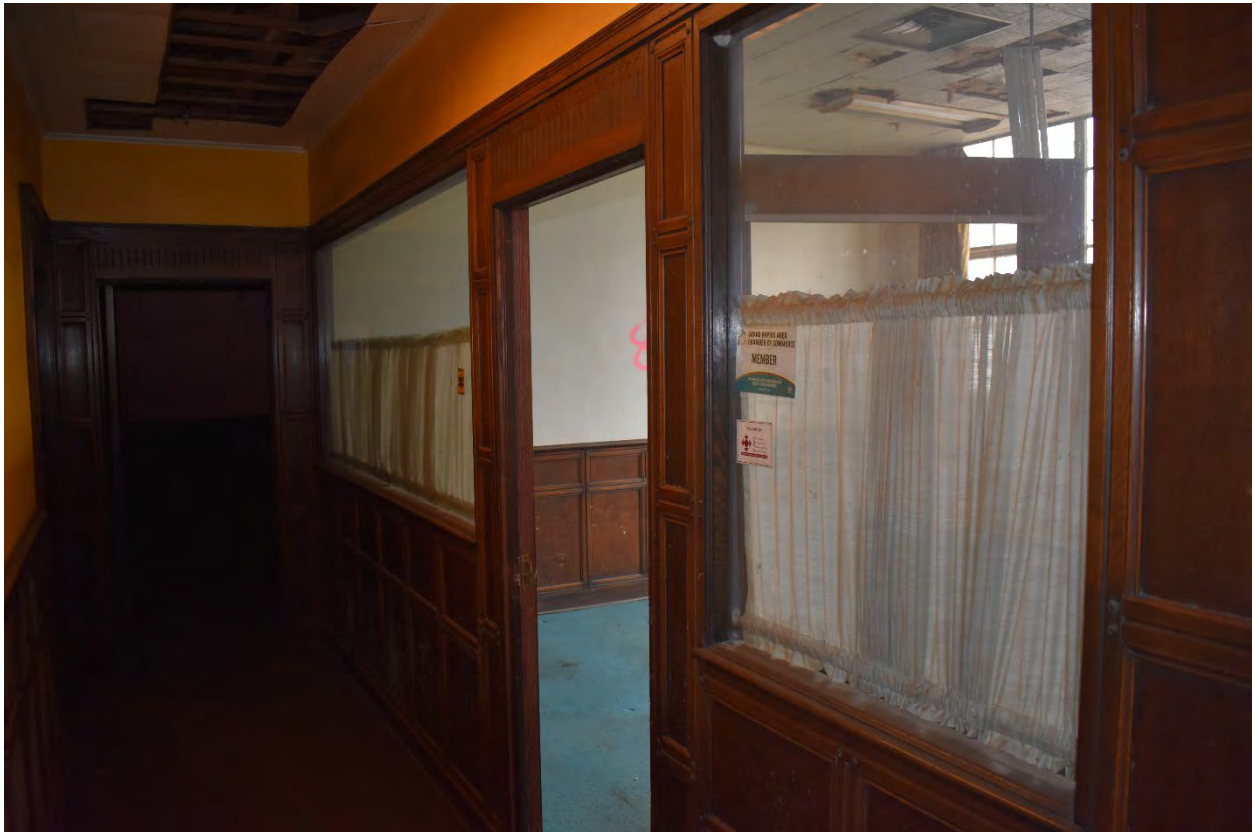
Interior view of the 5-Story Building
