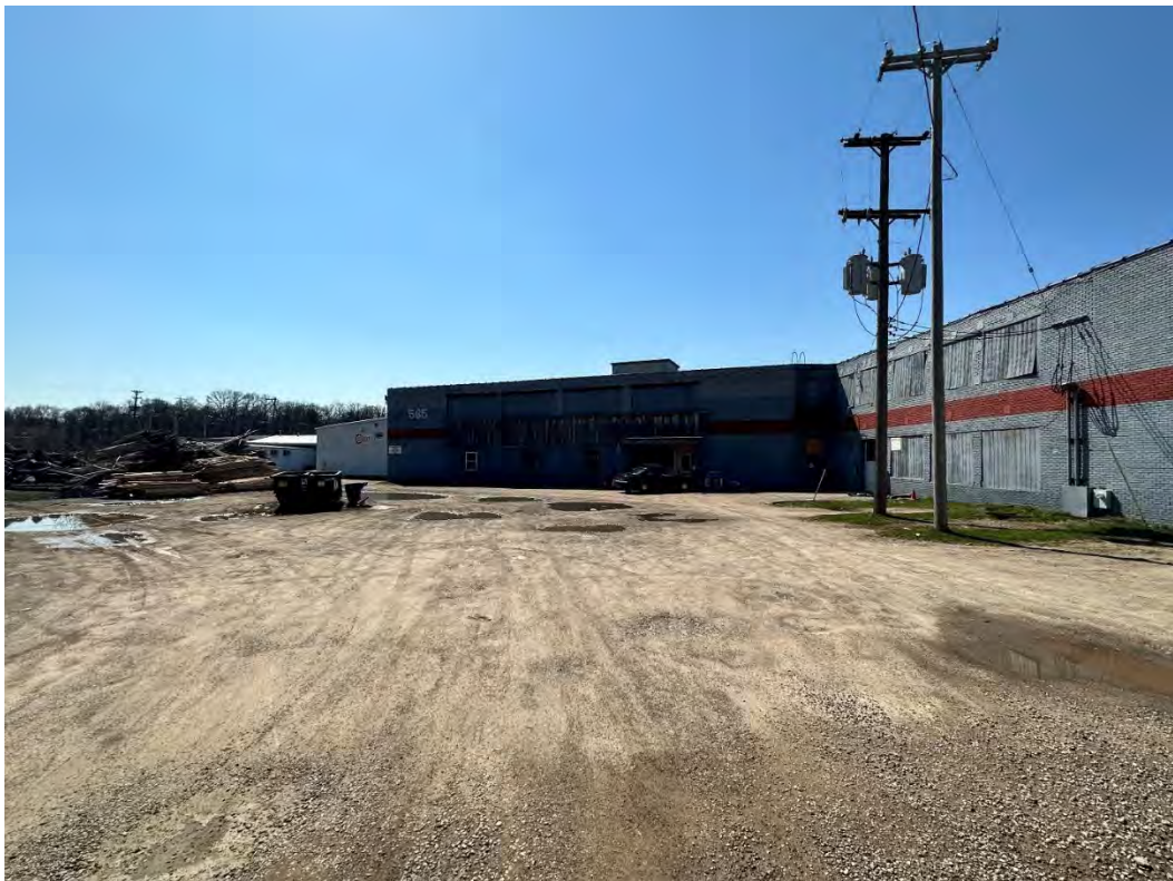
View looking west toward the North Commercial Site
