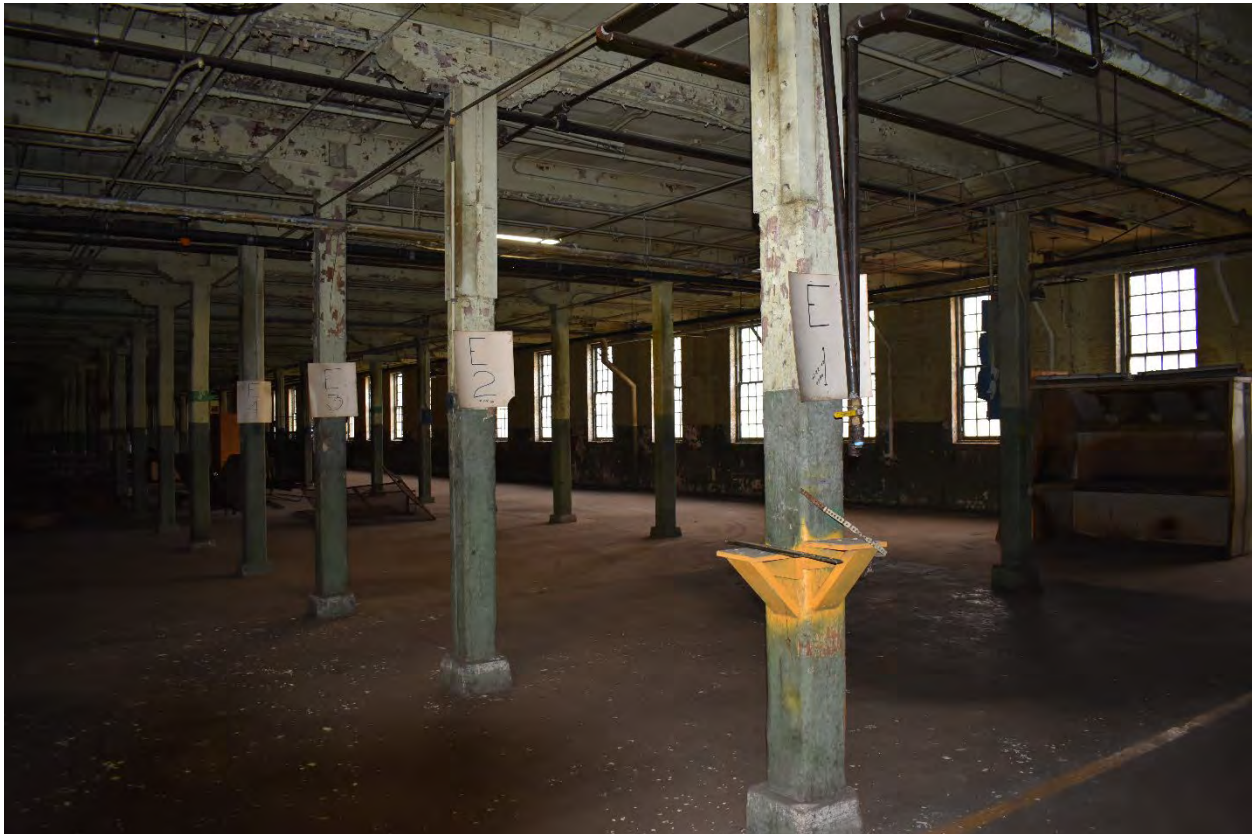
Interior view of the 3-Story Building
