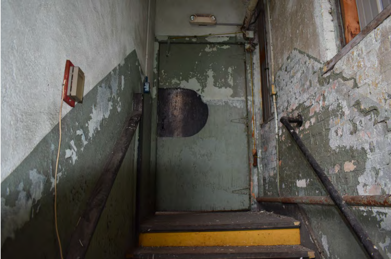
Interior view of the 3-Story Building
