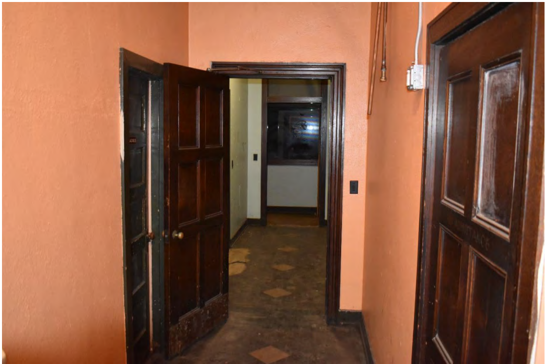
Interior view of the 5-Story Building
