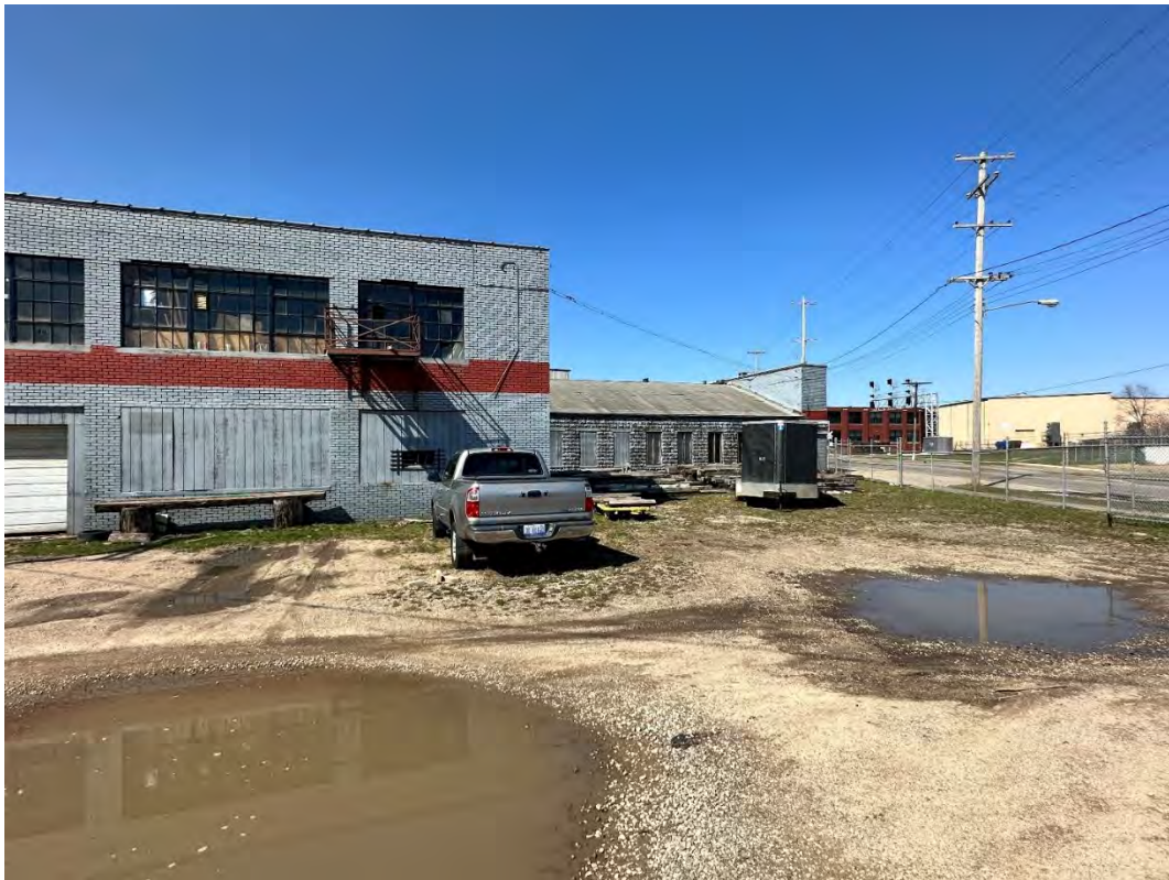
Looking North at a Portion of the existing buildings on the North Commercial site.
