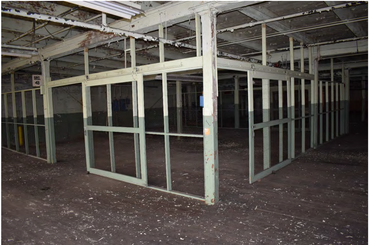
Interior view of the 3-Story Building
