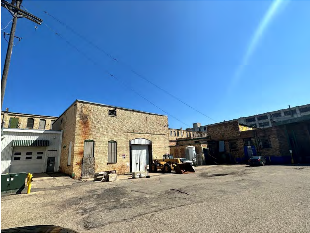
Looking West at the Boiler House Building
