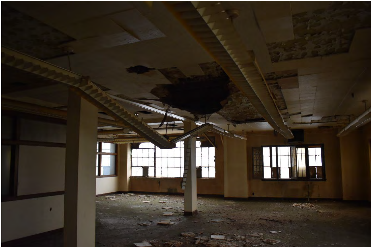
Interior view of the 5-Story Building
