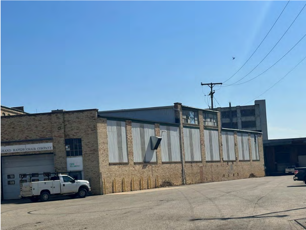
Looking SE from the west side of the Three-Story building
