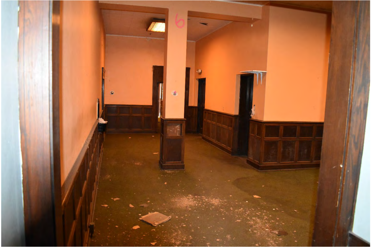
Interior view of the 5-Story Building
