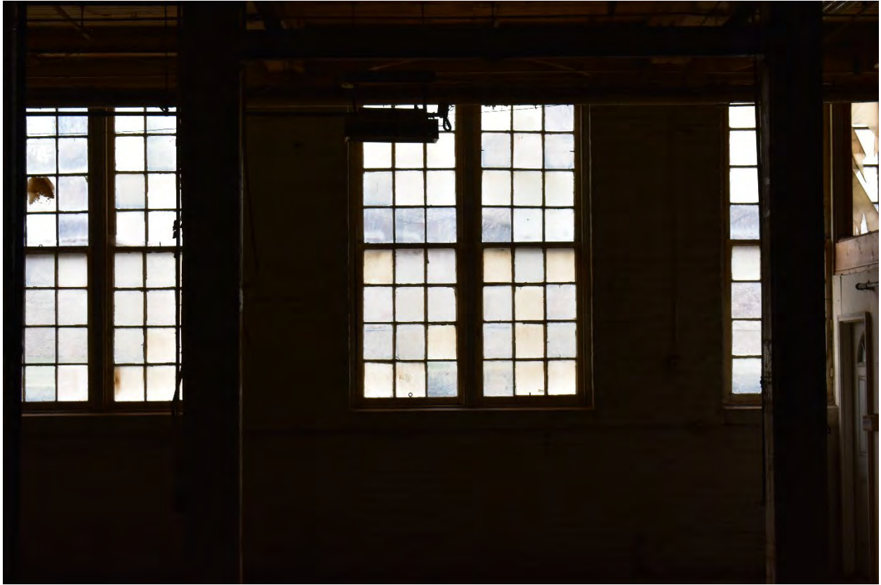
Interior view of the 3-Story Building
