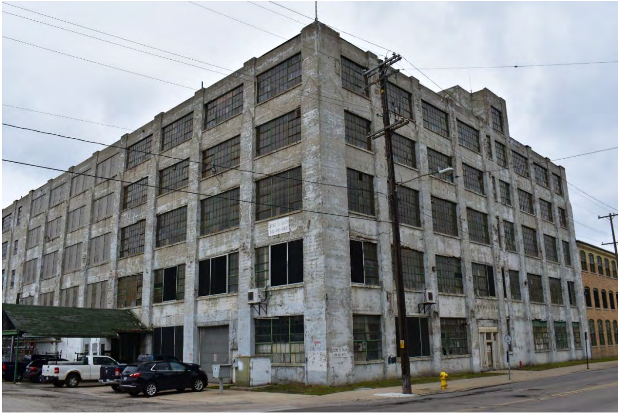
5-Story Building Looking NW
