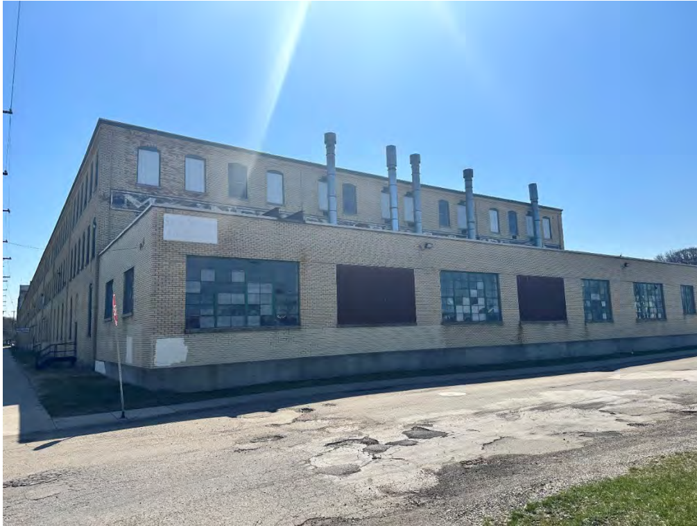
Looking South toward the Docks section of the three-story building
