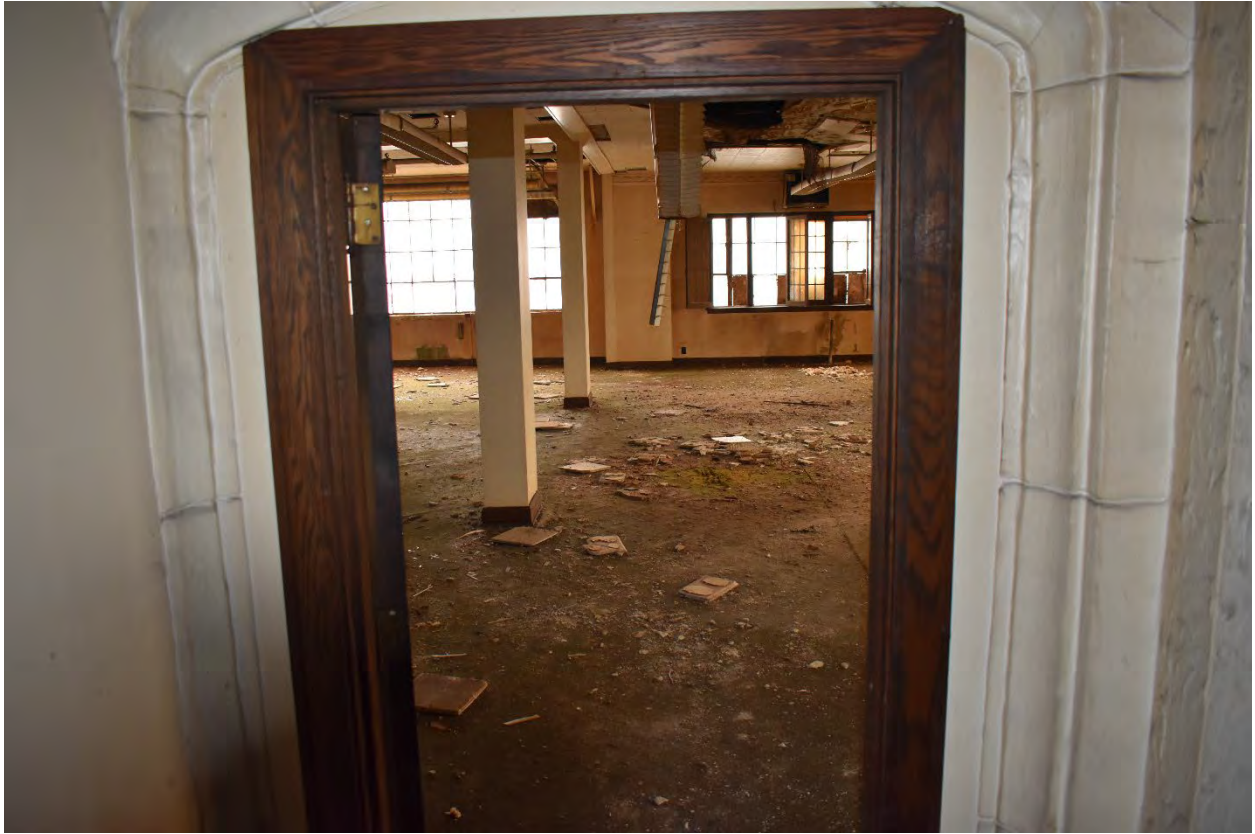
Interior view of the 5-Story Building
