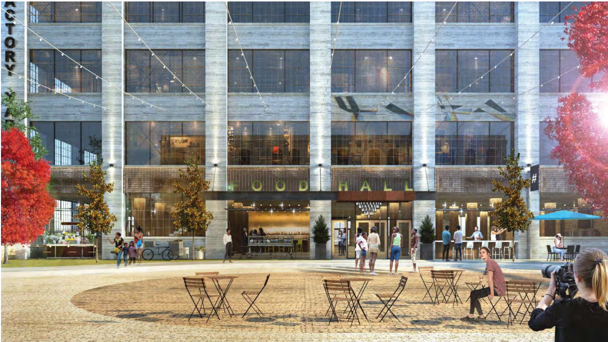
Facing South Toward the 5-Story Building from the Public Plaza
