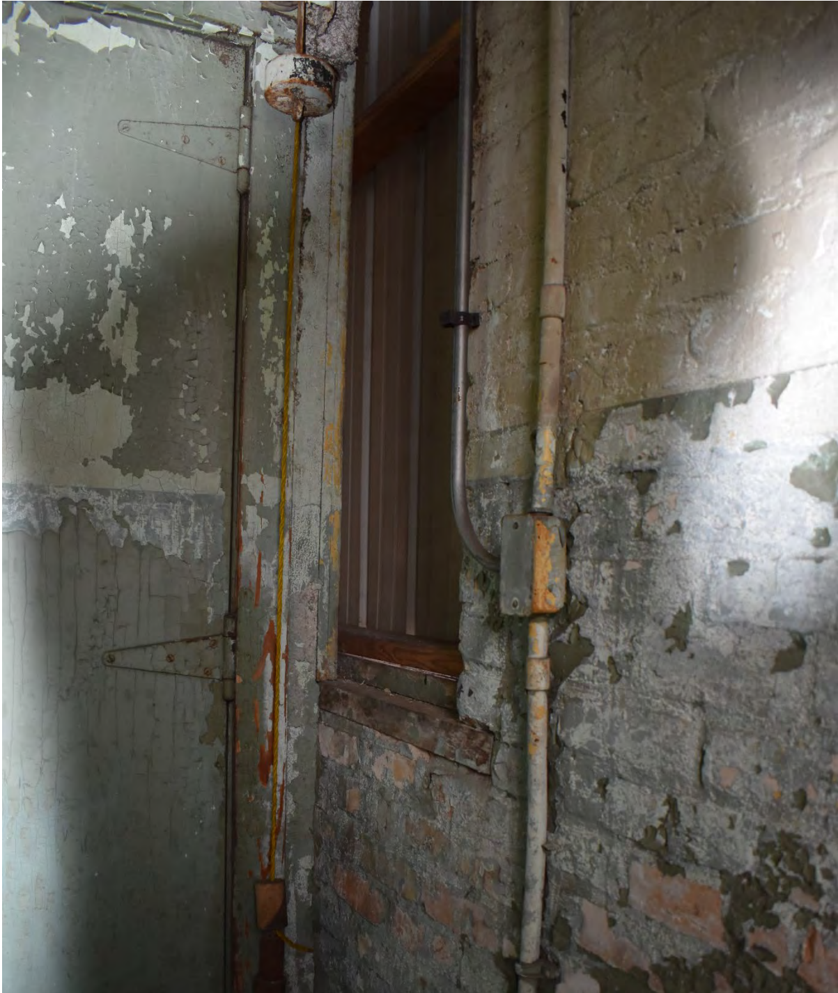
Interior view of the 3-Story Building
