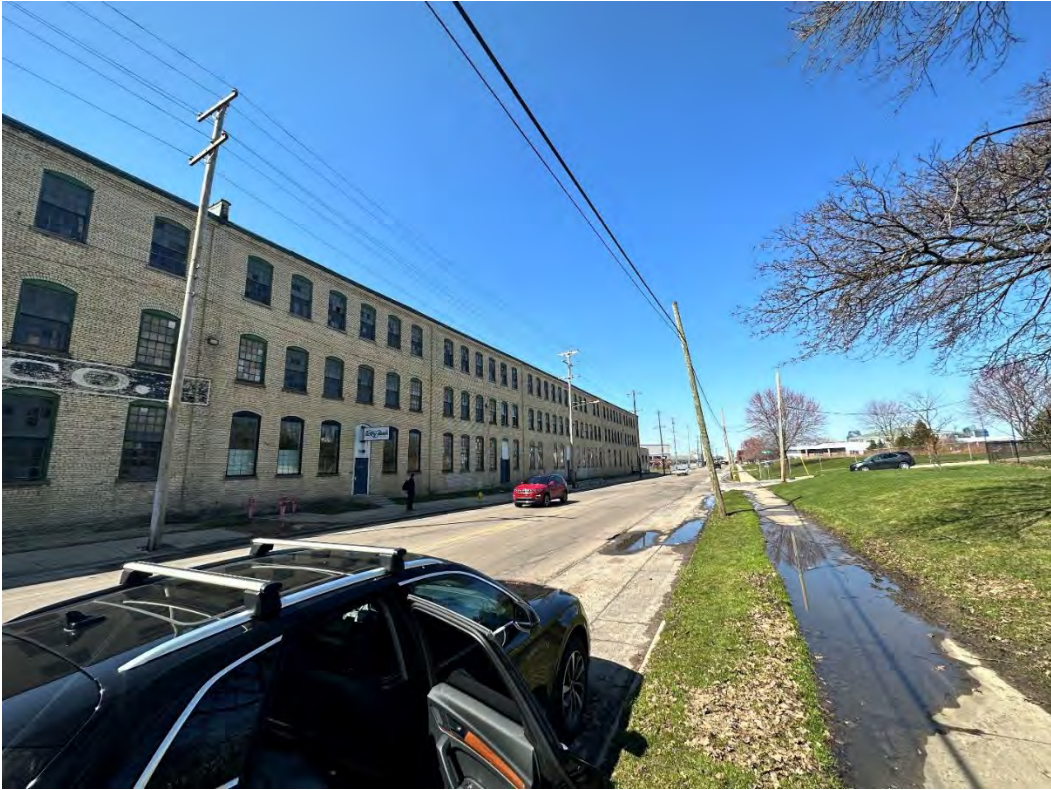
Looking NW at the 3-Story Building along Godfrey Avenue SW
