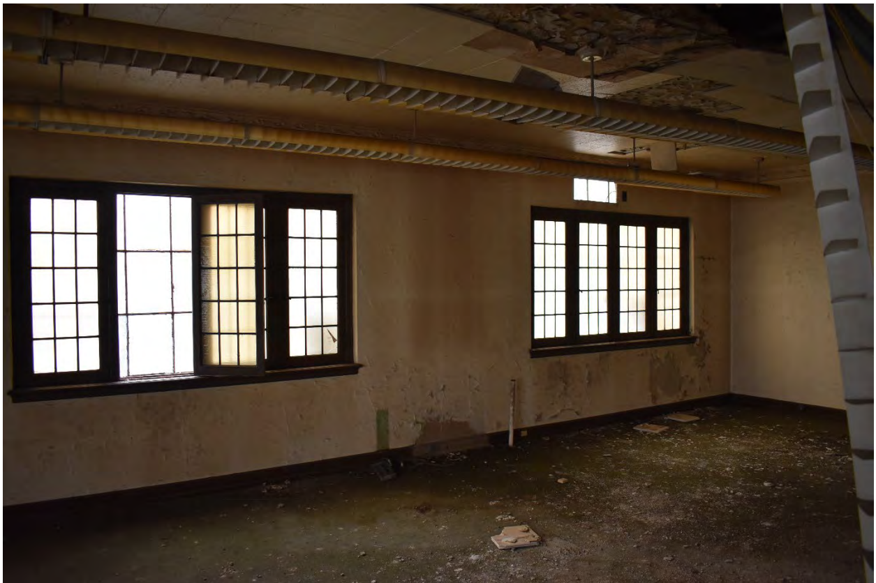
Interior view of the 5-Story Building
