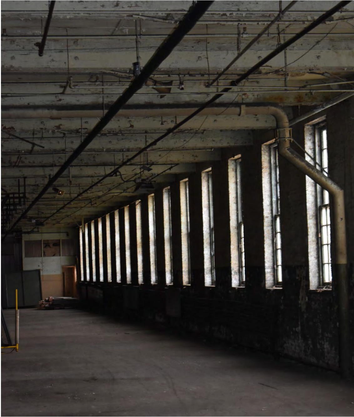
Interior view of the 3-Story Building
